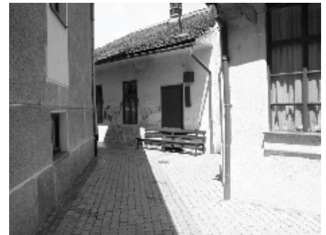
Auxiliary building needing renovation
