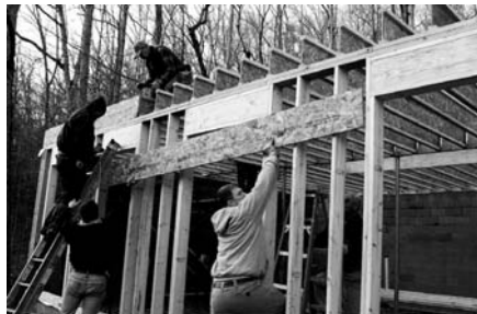
Rebuilding in Nashville, TN
