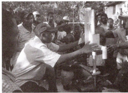
Initial installation of the pump on a new well
