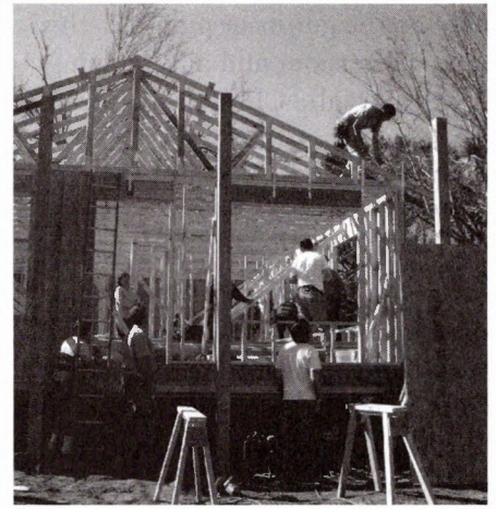
Katrina Work Team
