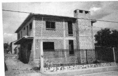
Guesthouse under construction
