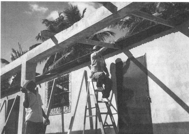
Working on a roofing project
