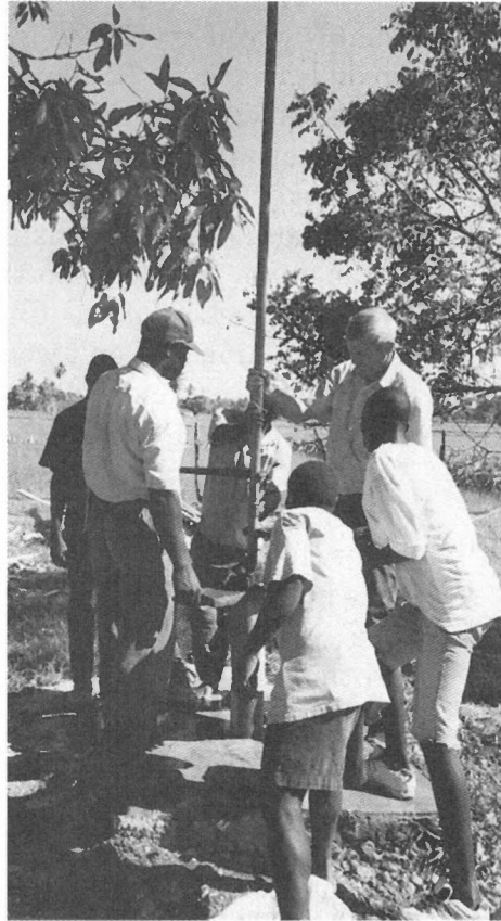
Finishing the installation of a well
